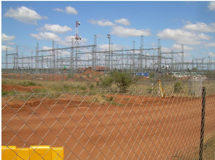
**Figure 3.4:** Photograph of a Substation, which transforms electricity from high to low voltage for consumer use.
