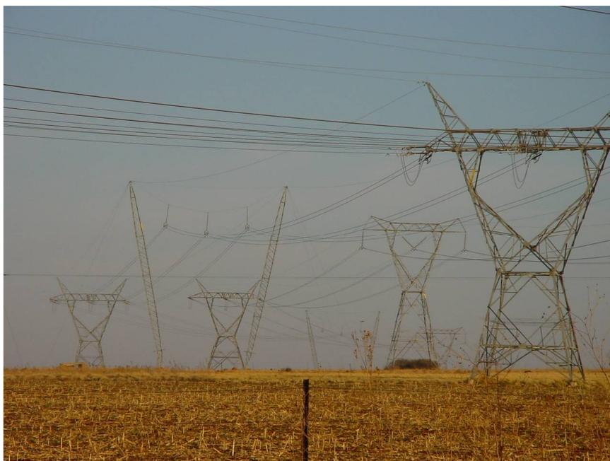
**Figure 3.2:** Photograph of Self-supporting Strain tower (in foreground) and Cross Rope Suspension tower (in centre) designs.
